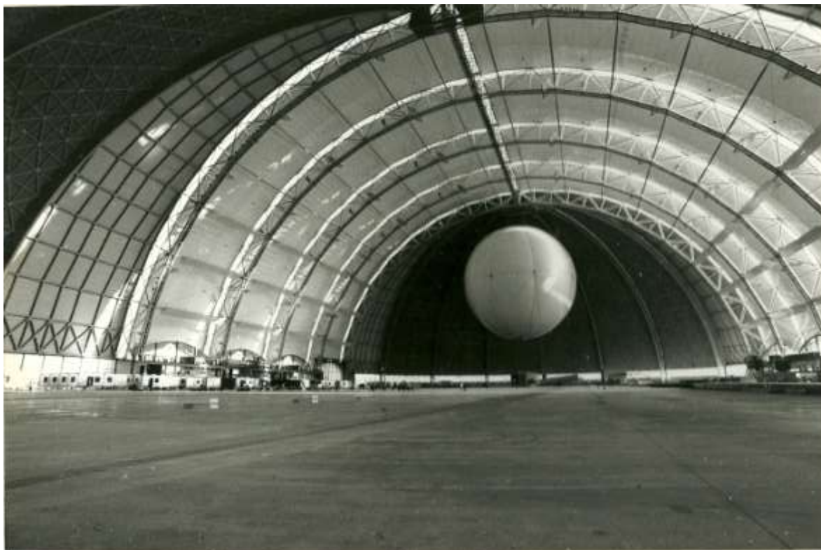
Cargolifter Hangar Brand. 2001.
